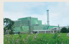
Municipal waste incineration Taiwan
