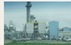
Coal fired boiler Canada
