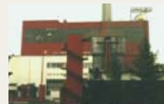
Coal fired boiler Czech Republic
