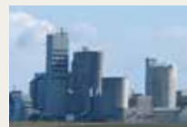
Cement plant Austria
