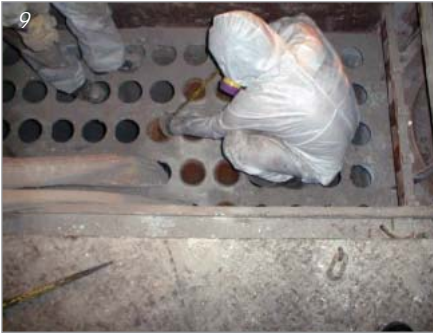
Figure 9. Baghouse inspection.
