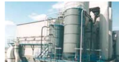
Increased dust emissions are an absolute disaster for a WTE plant. Inhomogeneous fuel quality requires a highly flexible flue gas treatment system, including the bag filter unit being the barrier for all solid substances.
